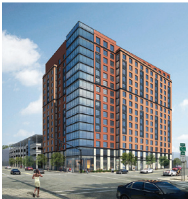
Photo: Bluestone Organization. Photo: ICF Panels, Inc.
